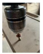
6. Make marks on the wall – copy them froms left side (inside), copy them from right side (outside): those will be the centers for drill holes, drill (with 12mm drill) holes 60mm deep, hit in plastic dowel, use screw A4 with electric screw driver, in the finish use wrench 13mm to screw the nut.
